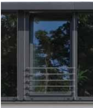
Metal balustrades add style and balance
