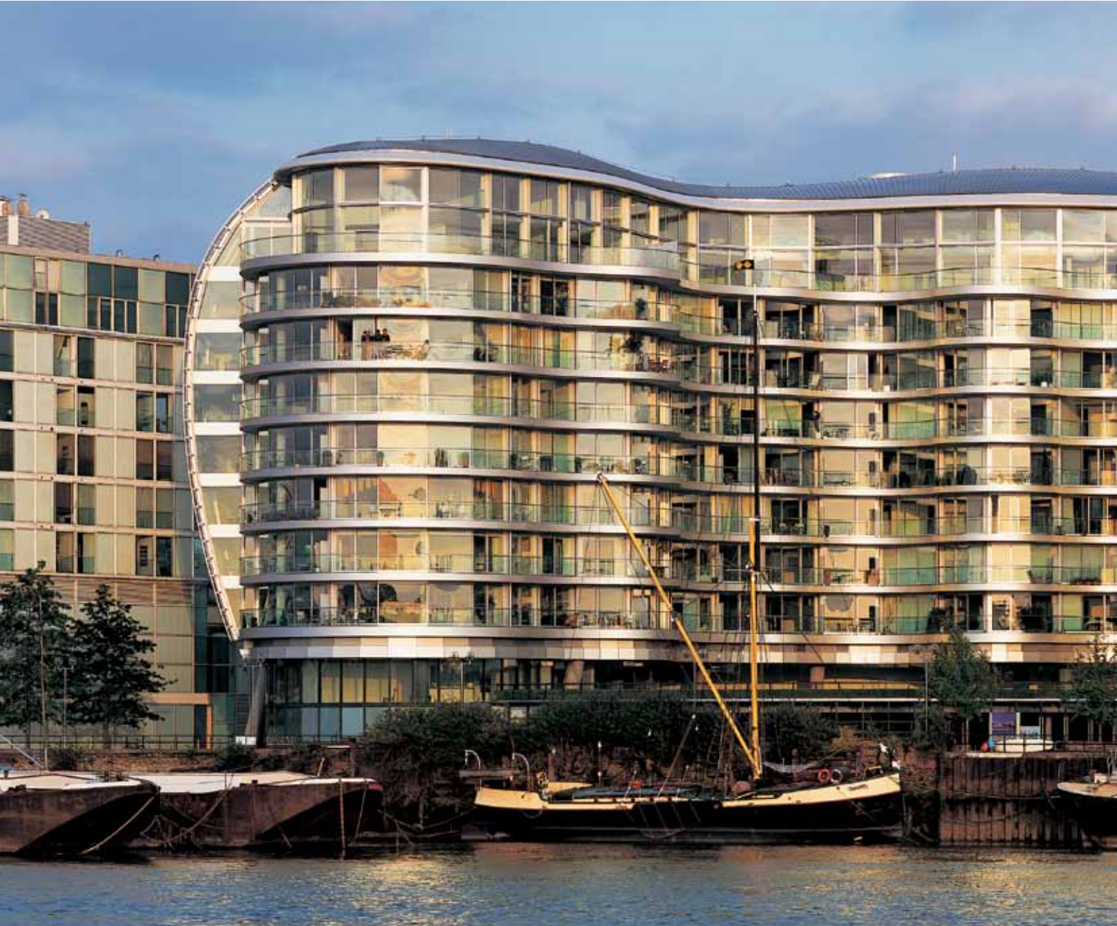
Albion Riverside, London, designed by international architects Foster + Partners and featuring Schueco systems
